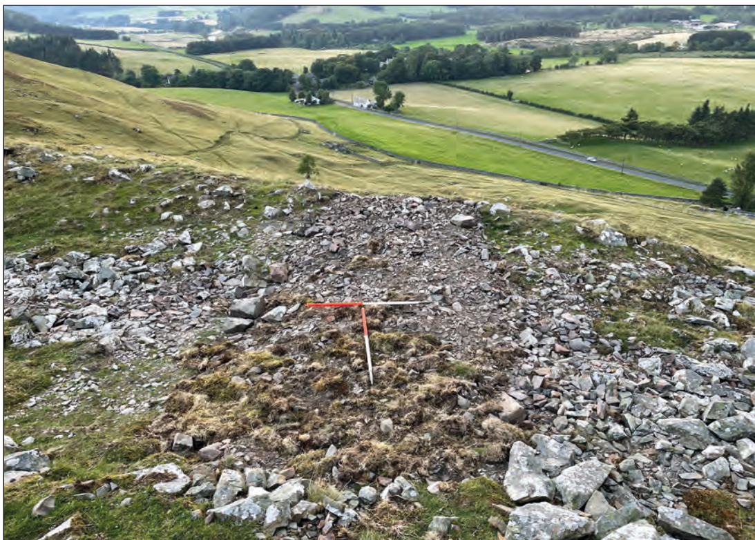
Plate 31: Backfilled Trench 3 (20 September 2022)
