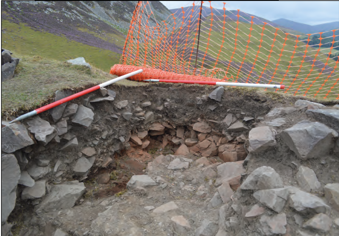
Plate 14: Burnt and discoloured rampart core (2010) from NE
