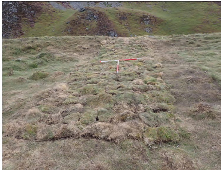
Plate 26: Backfilled Trench 1 (19 August 2022)
